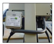
Mini-meter installed on the back of a Level-2 charging station to record kWh usage. Photo courtesy: Charles Whalen
