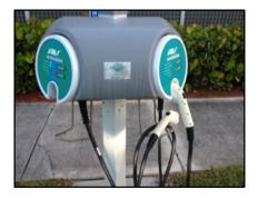
A Level-2 Charging Station (dual unit) with a standard cord set, carelessly stored by a user. This can create a tripping hazard, or allow rainwater to enter the connector – prematurely aging the equipment. Photo credit: Brian Hanrahan, Florida Power & Light Co.
