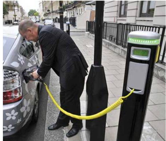
On-street charging near end of block.
