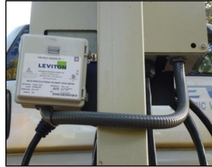
Mini-meter installed on the back of a Level-2 charging station to record kWh usage. Photo courtesy: Charles Whalen
