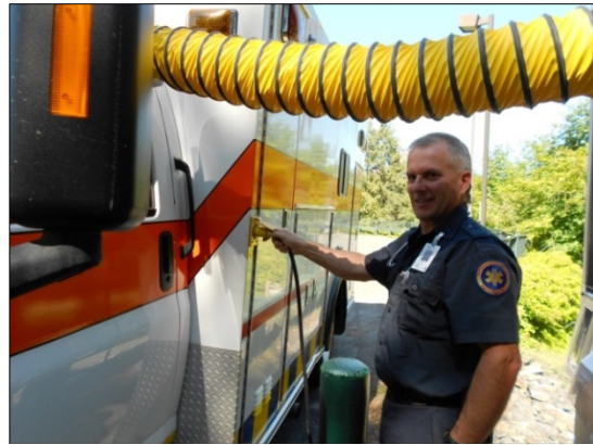
Figure 3.2. Ambulance hooked up to a MediDock for power and conditioned air. (Photo courtesy of Craufurd Manufacturing)
