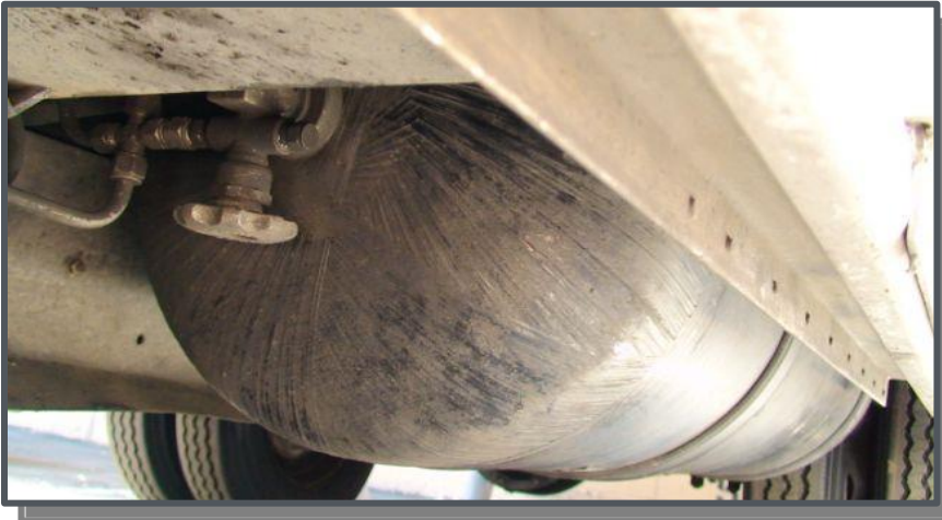
No shielding of exposed cylinder under vehicle – this dome failed
