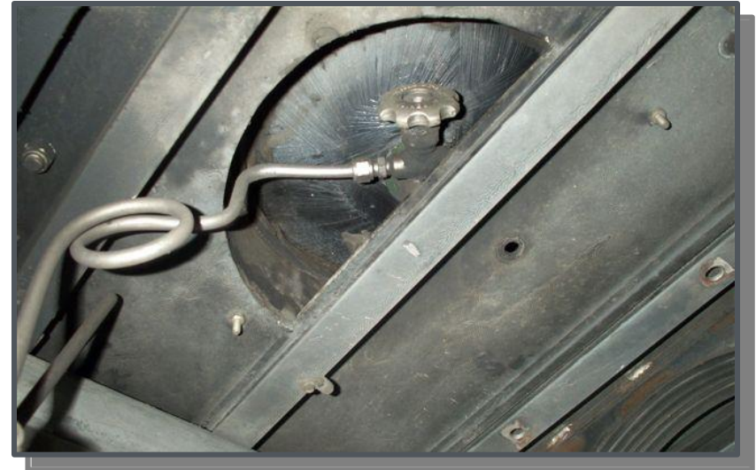
Cylinder improperly mounted on steel ring
