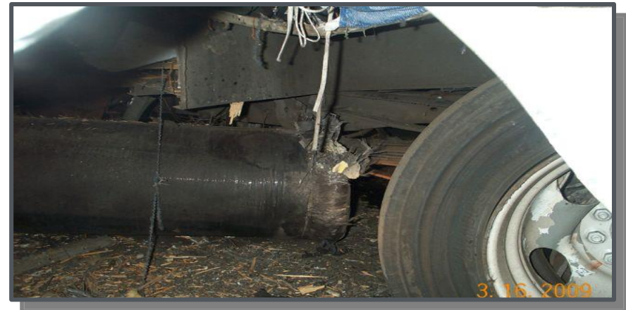
Dome of under mount cylinder failed
